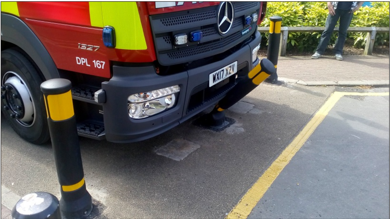
Photograph 5 – collapsible bollard for fire access.
