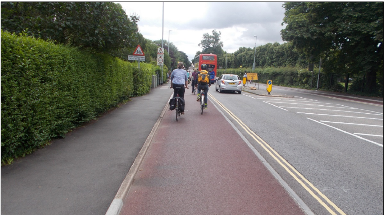
Photograph 8 – red asphalt used for a stepped cycle track, Hills Road, Cambridge.
