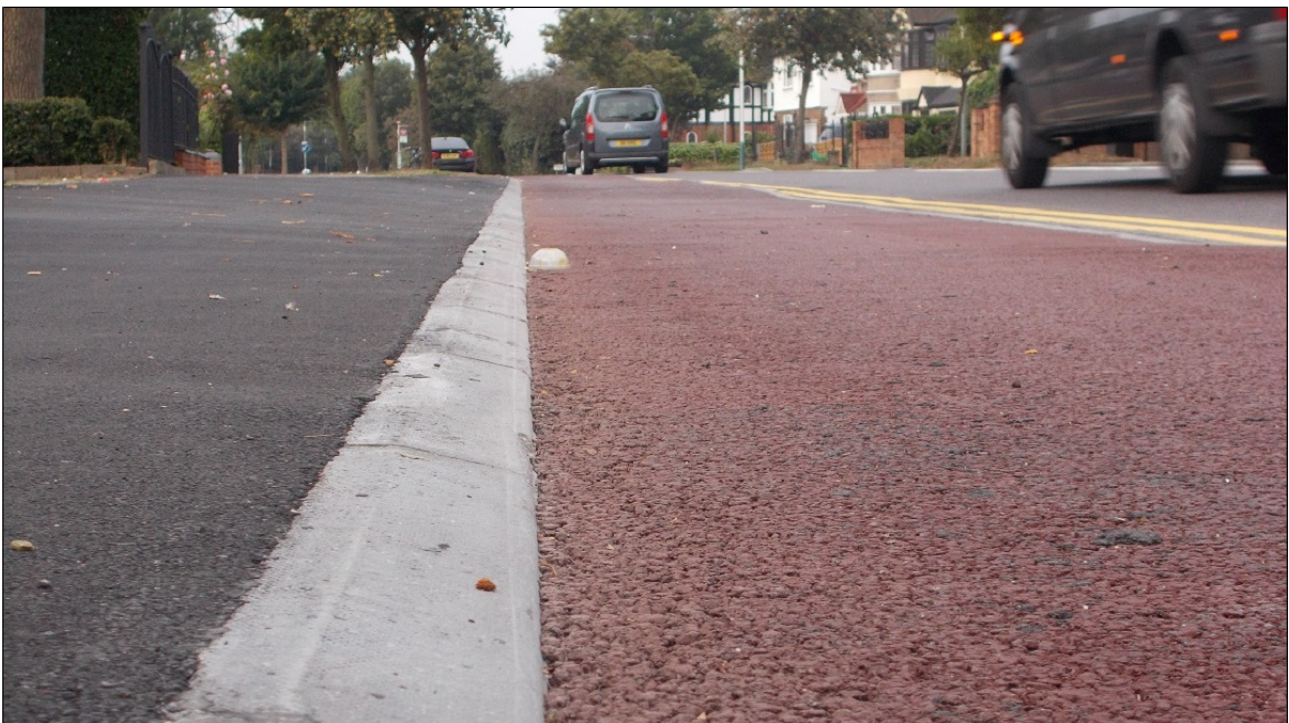
Photograph 2 – forgiving kerb between cycle track and footway, Main Road, Romford.
