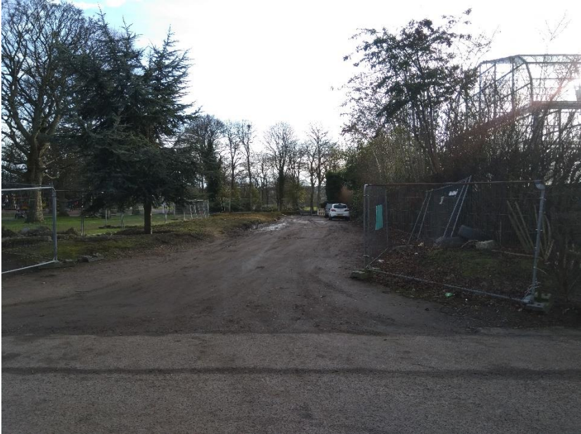
Figure 13: Temporary (?) access road east of Winter Gardens
